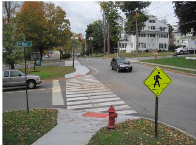
Figure 6 - Pedestrian accommodation at Elm Street
