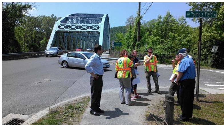
Figure 25 – Young's Field Road look west along Bridge St.
