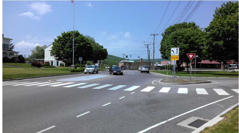
Figure 24 – East Main Street intersection (looking west along Bridge St.)
