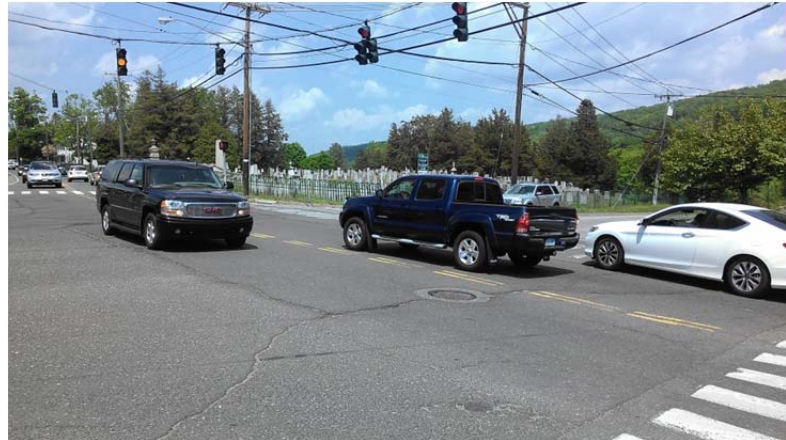
Figure 27 – East Street/Elm Street intersections (looking north)
