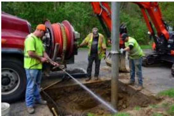
Catch Basin repair
