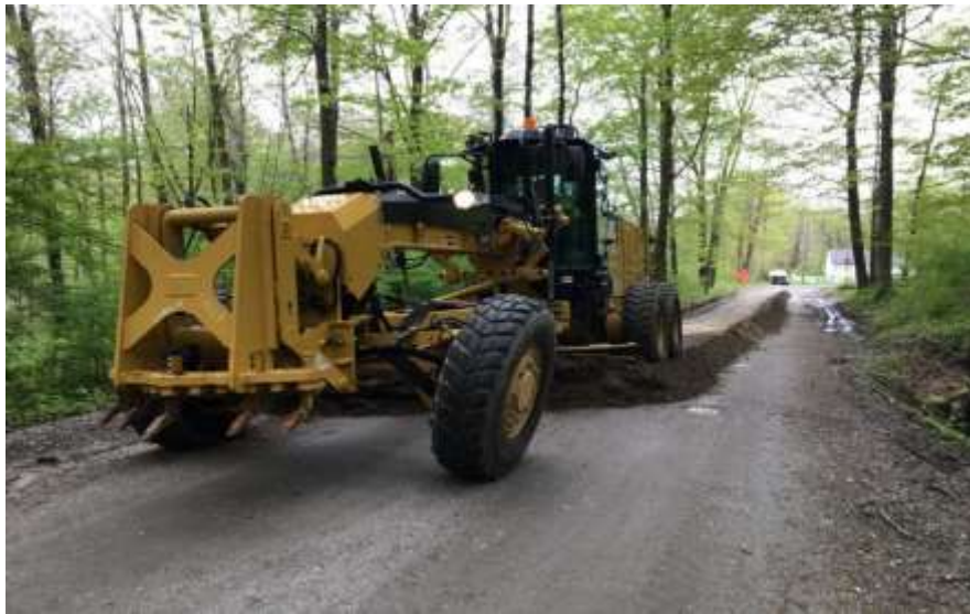
Dirt road grading
