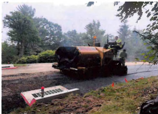
Repaving Mockingbird Lane
