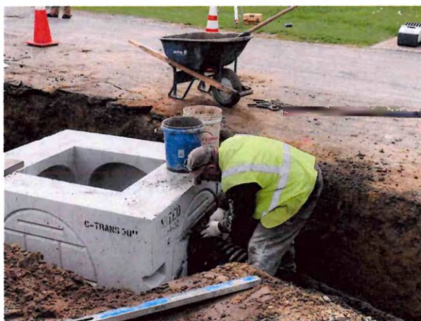
Bostwick Place Drainage
