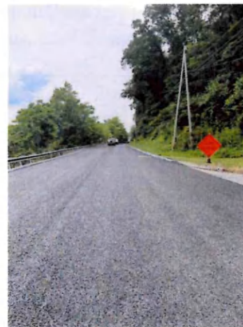
Double Chip seal on Grove Street
