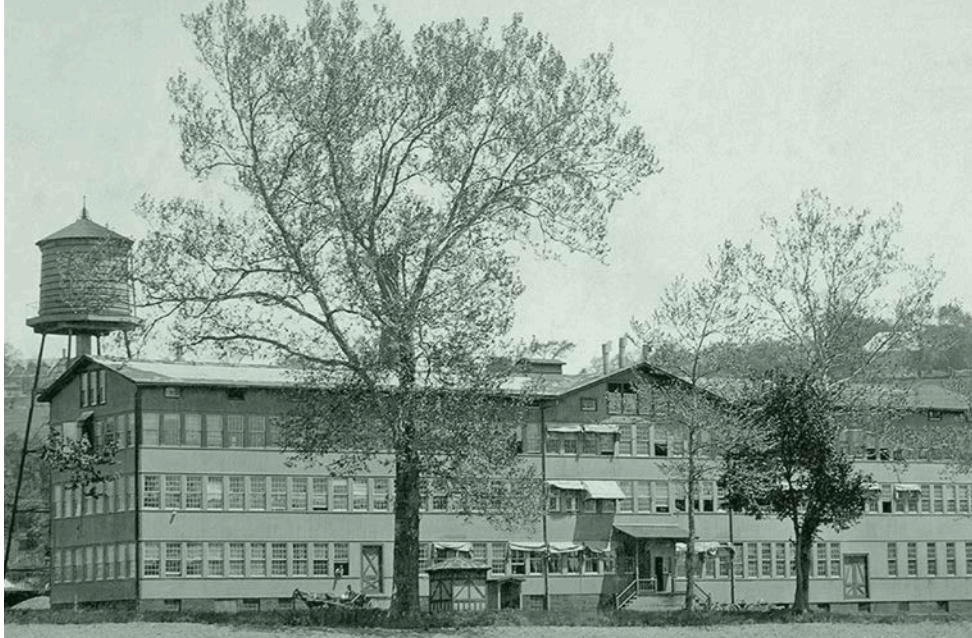
NEW MILFORD HAT FACTORY.
