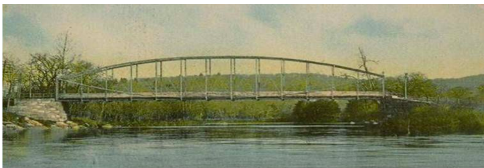
BOARDMANS BRIDGE, C. 1913.
