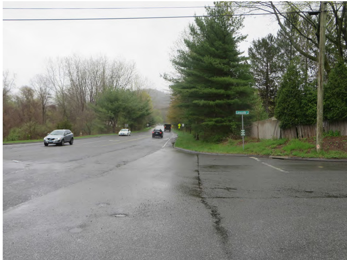
Photograph S15: Still River Drive facing west from intersection with Lanesville Road, at right.
