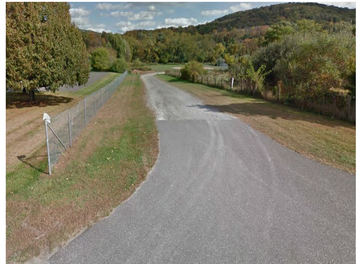
Photograph S14: Gravel road, facing east downhill from Pickett District Road to Town owned ballfields and potential route of trail.
