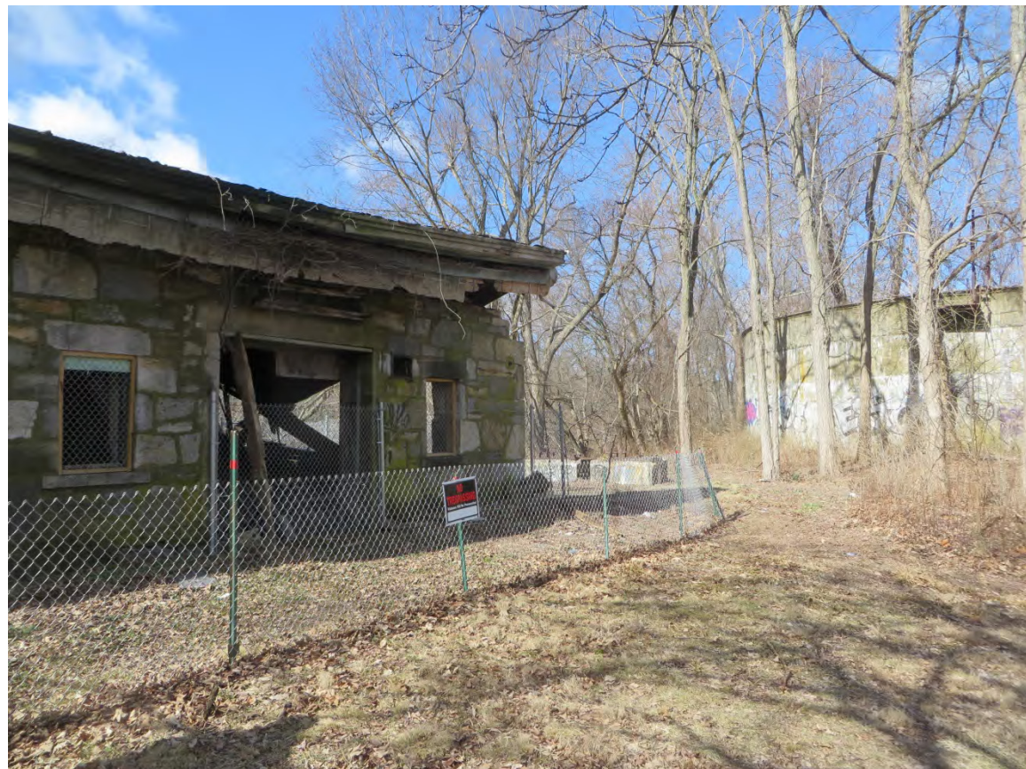
Photograph S8: East façade of old granite and fieldstone mill building in Hidden Treasures Park, with storage tank to the north.
