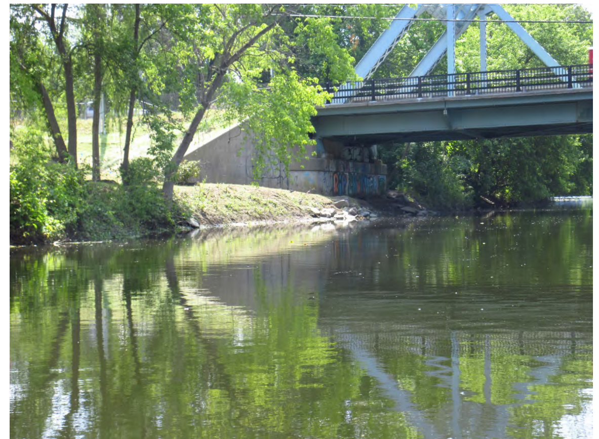
Photograph S6: Potential route of trail beneath the east side of the Bridge Street Bridge, immediately adjacent to the Housatonic River, facing southeast.
