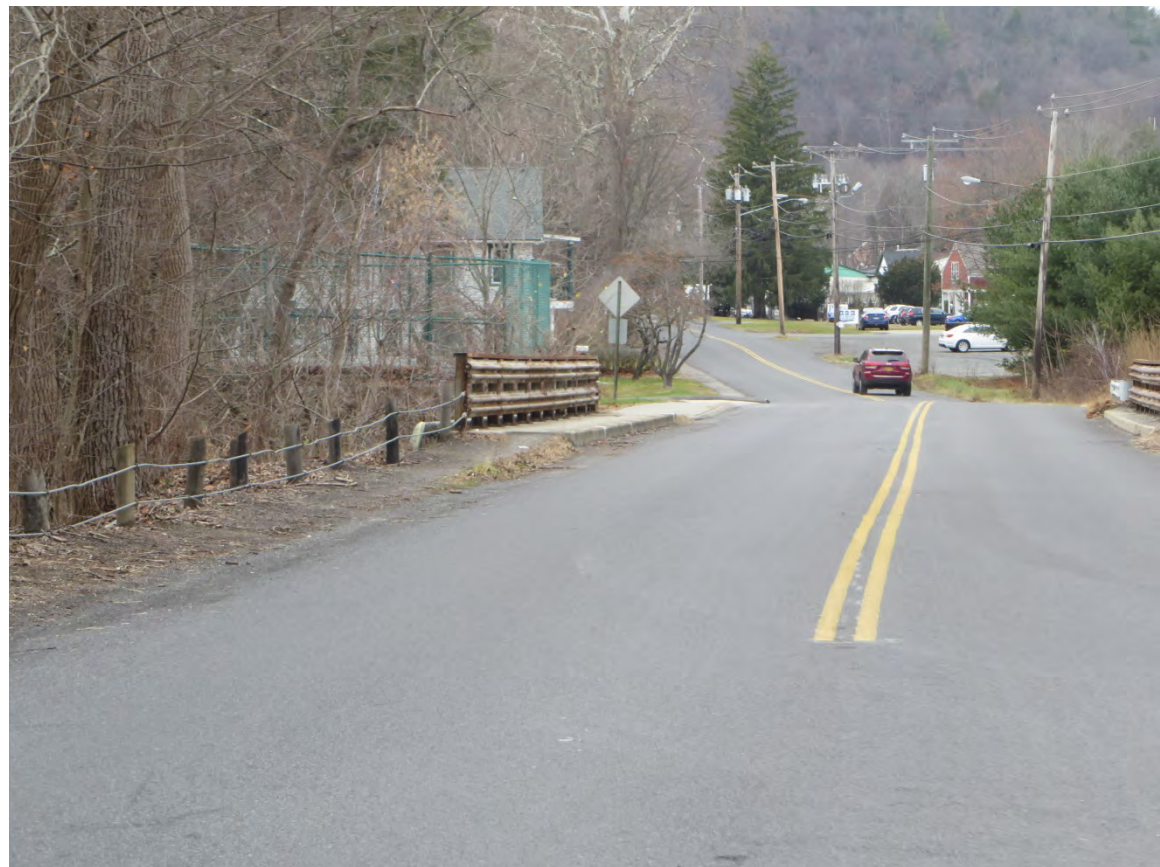
Photograph N22: Facing northwest from the center of Housatonic Avenue toward a small bridge crossing over the West Aspetuck River.
