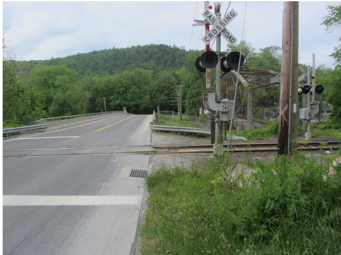
Photograph N1: Boardman Road facing east from north side of road to railroad tracks, with the existing Boardman Bridge at left and the historical 1888 wrought-iron, lenticular truss Boardman Bridge (National Register of Historic Places) at right.
