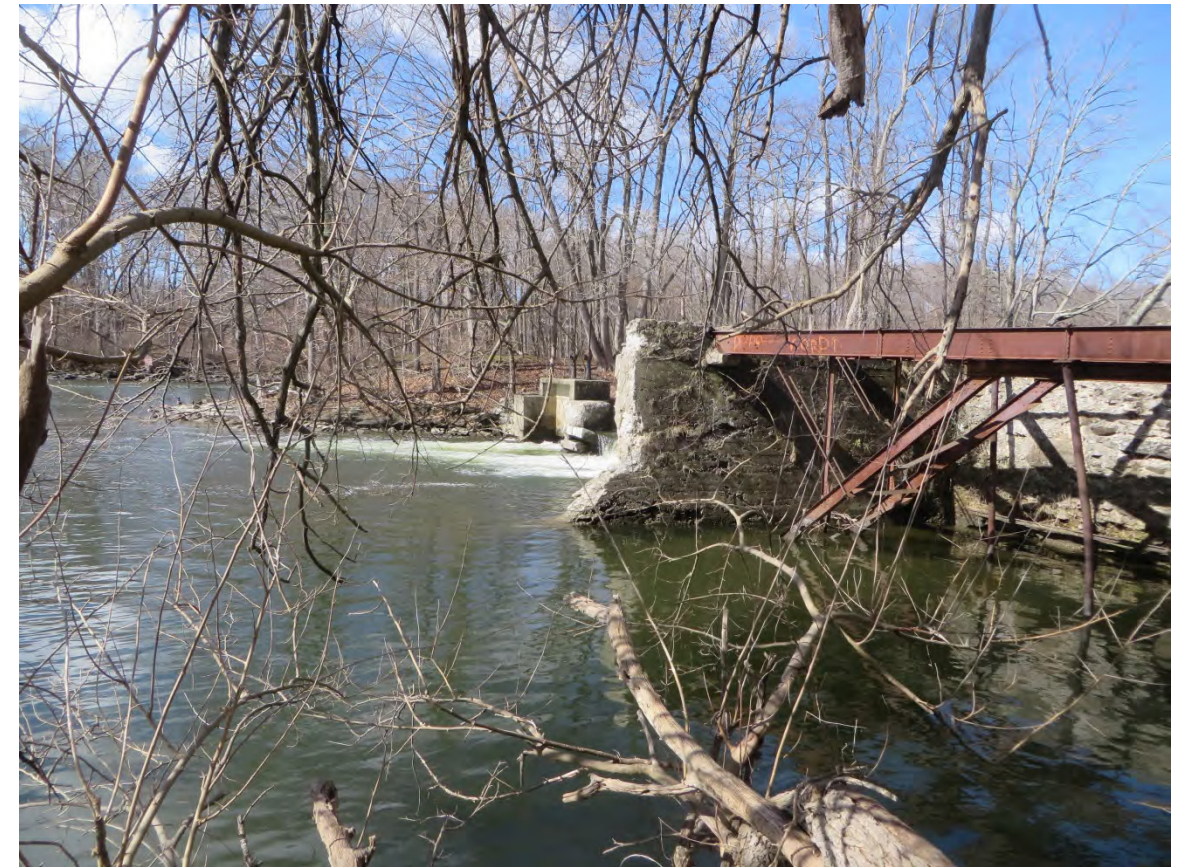
Photograph S9: Remains of eastern portion of Bleachery Dam adjacent to the mill building in Hidden Treasures Park, facing northwest.
