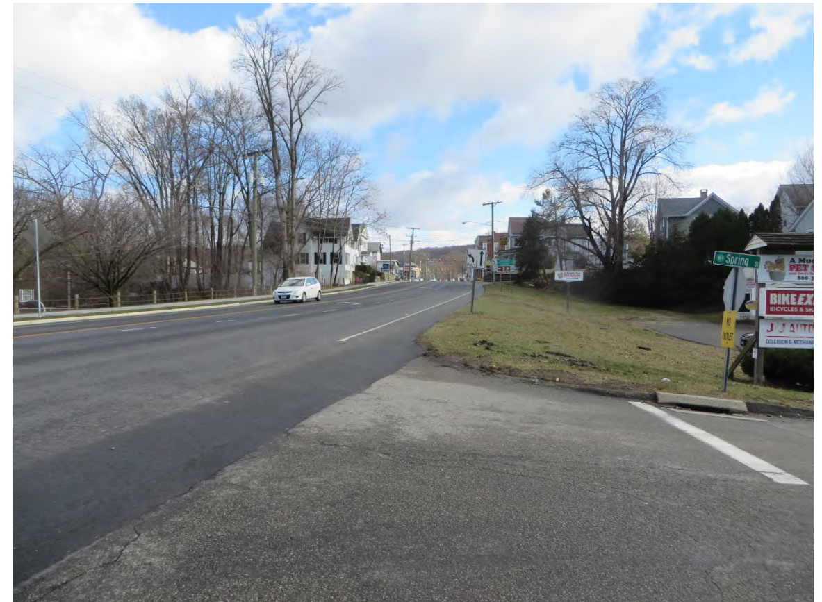
Photograph S5: South side of Bridge Street facing east from just west of Spring Street.
