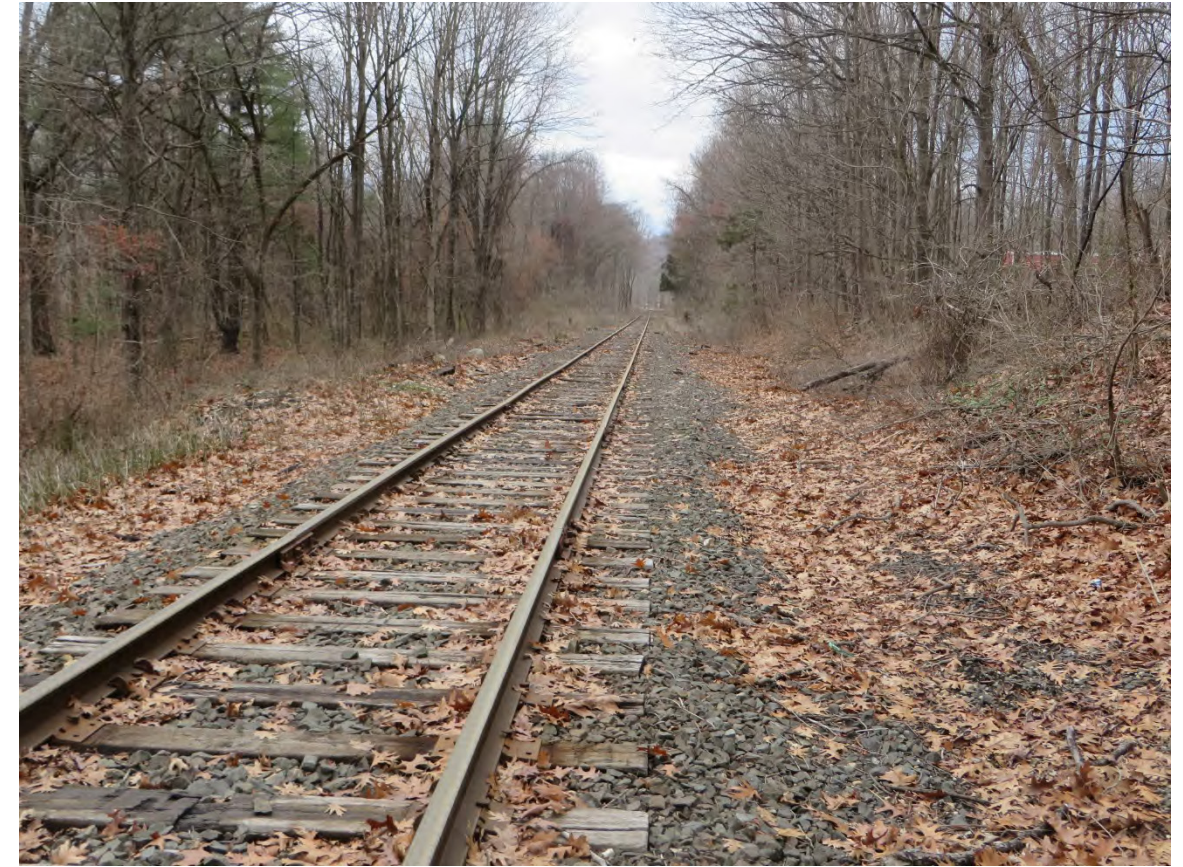
Photograph N7: Facing north to railroad cut into the terrain, with an embankment down at left, and an embankment up at right.
