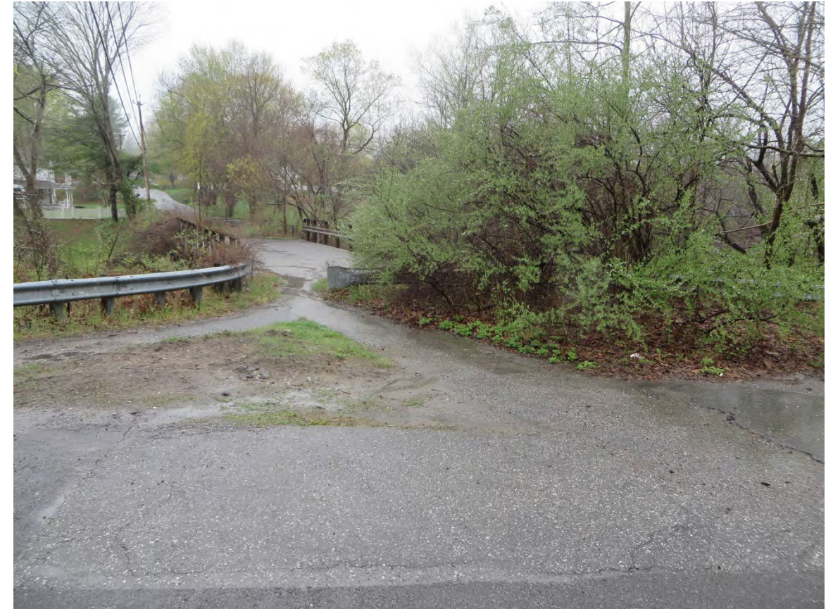
Photograph S21: Facing southwest to the Lanesville Road Bridge over the Still River at the south end of Frank's Lane and Harrybrooke Park's northern parking lot.
