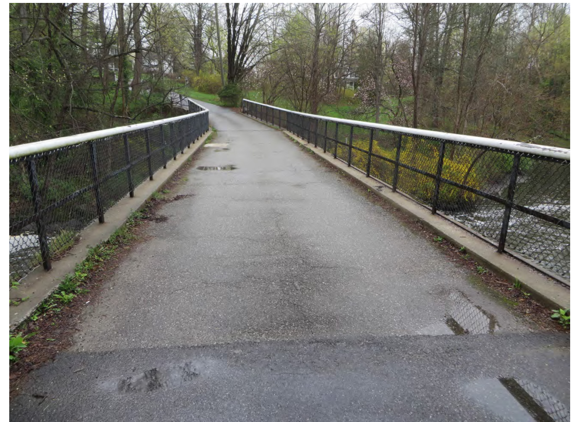
Photograph S22: Facing northwest to the existing Harrybrooke Park Bridge over the Still River that exits onto Lanesville Road.
