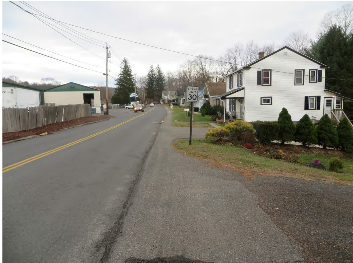
Photograph N21: Facing southeast on south side of Housatonic Avenue to alternative proposed route of the trail.
