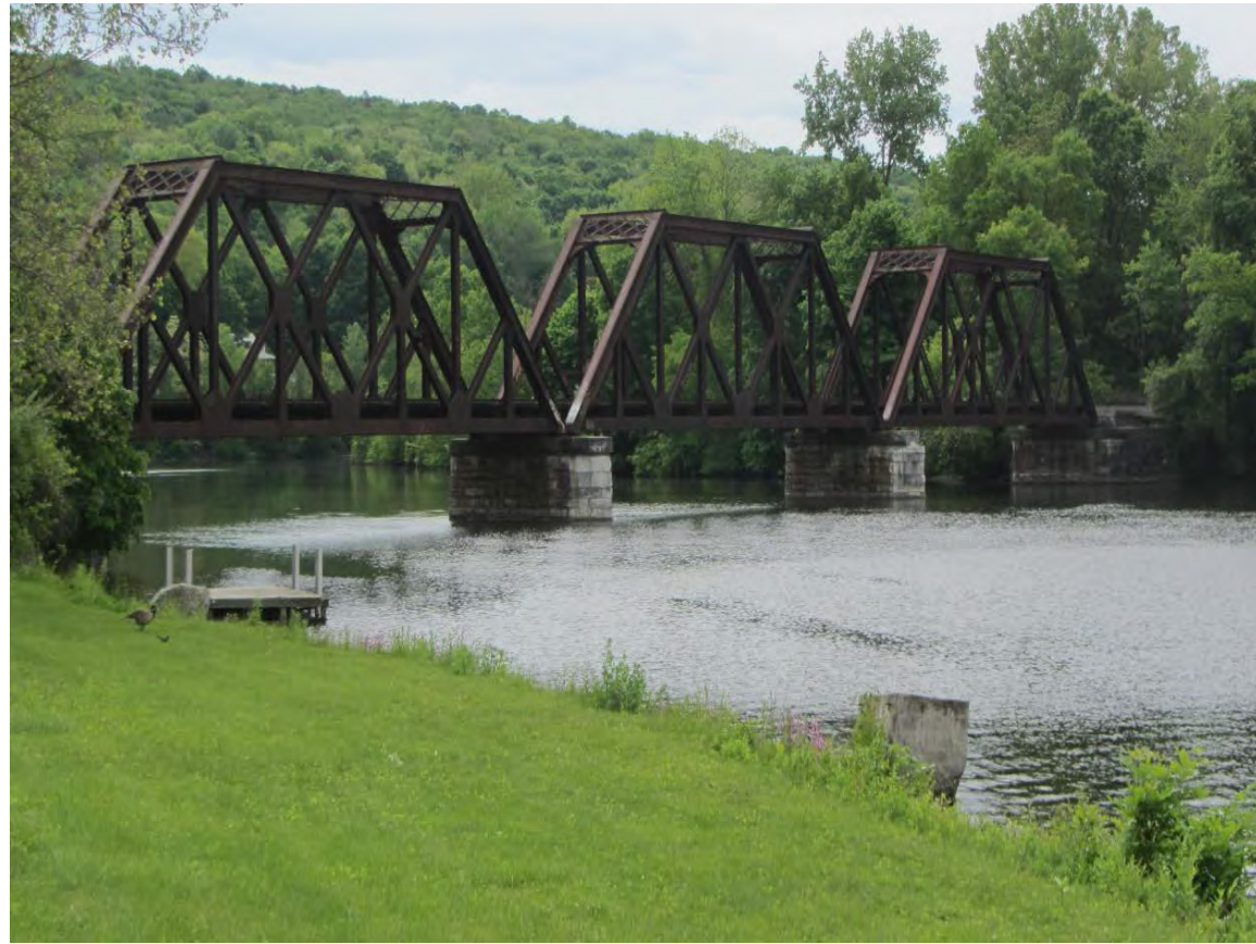
Photograph S11: Existing railroad bridge over the Housatonic River, south of the West Cove Marina property, facing south.
