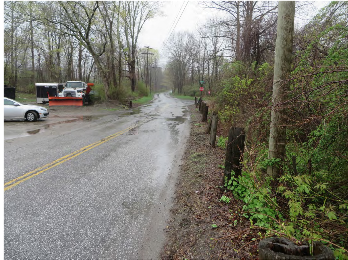
Photograph S23: Erickson Road just north of its intersection with Cross Road, facing south.
