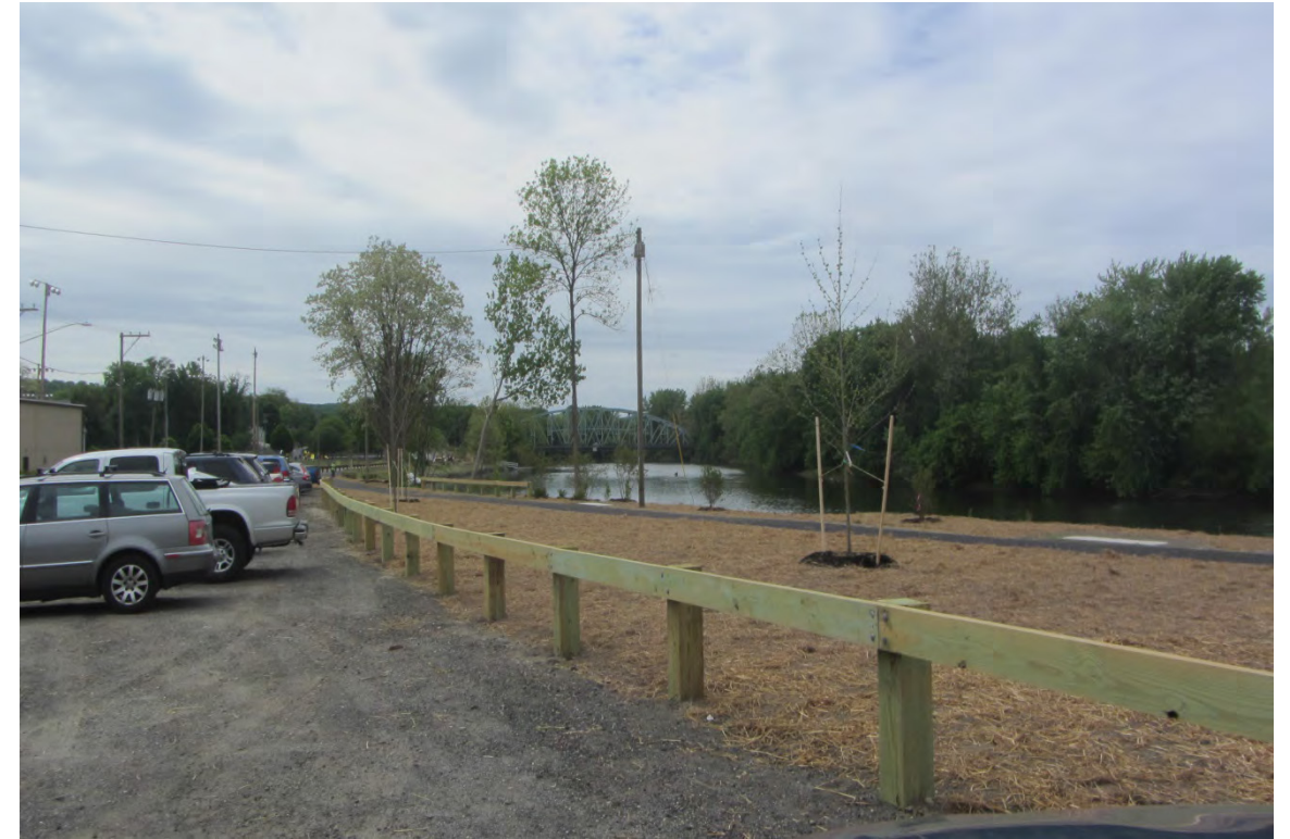
Photograph N19: Recently completed (June 2017) Riverwalk Park between Youngfield Road and the Housatonic River, facing south to the bridge at Bridge Street.
