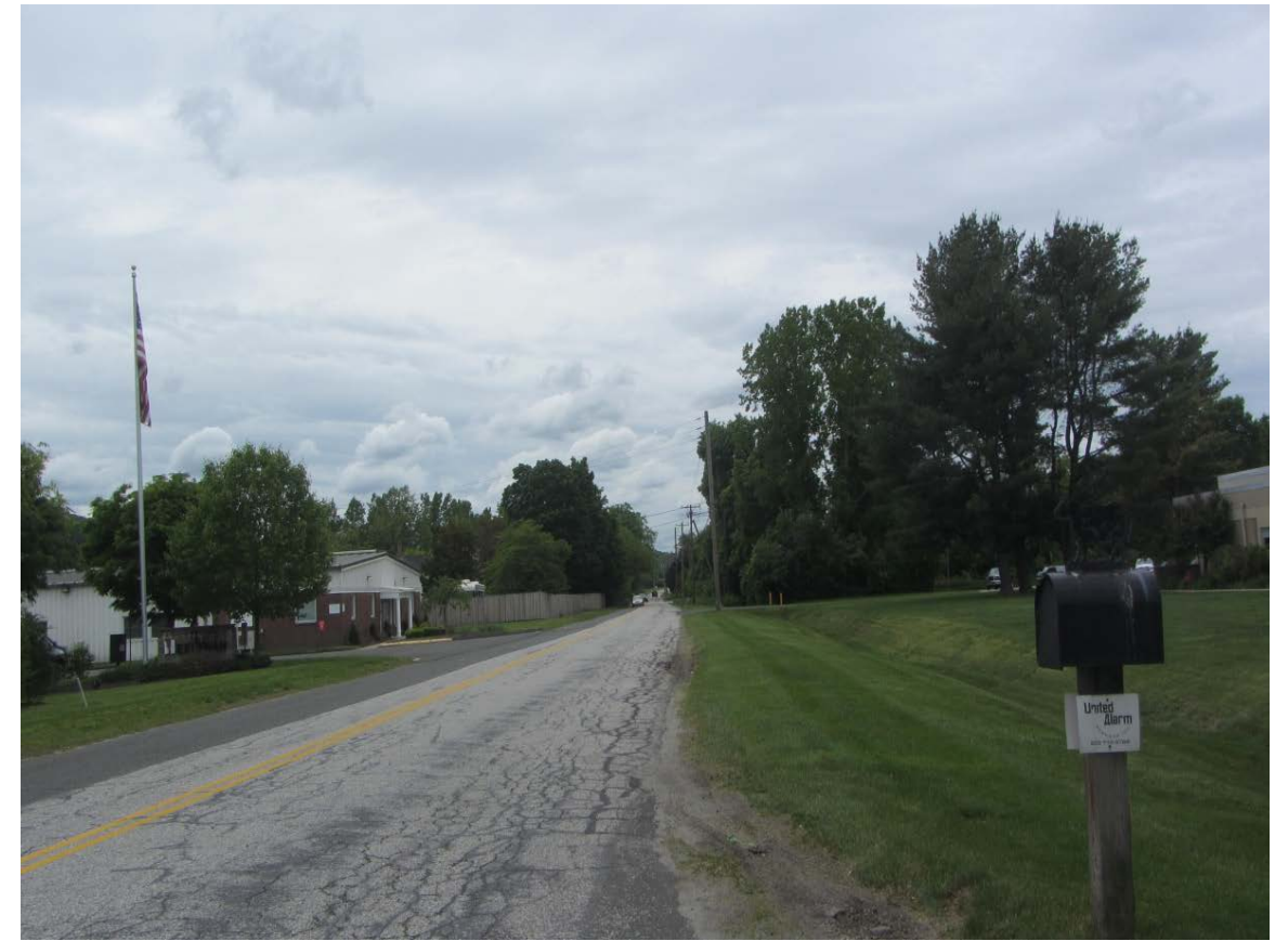
Photograph S13: Looking south on west side of Pickett District Road in front of Kimberly Clark toward 71 Pickett District Road.
