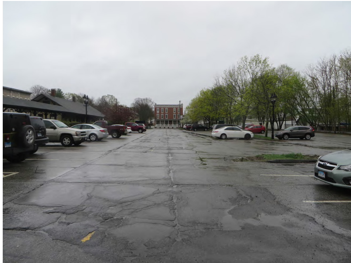
Photograph S3: Parking lot east of and elevated above Youngs Field, facing south to Bridge Street.
