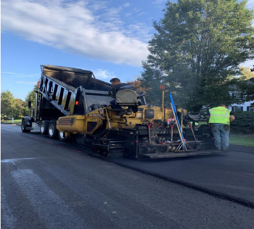
Paving top course
