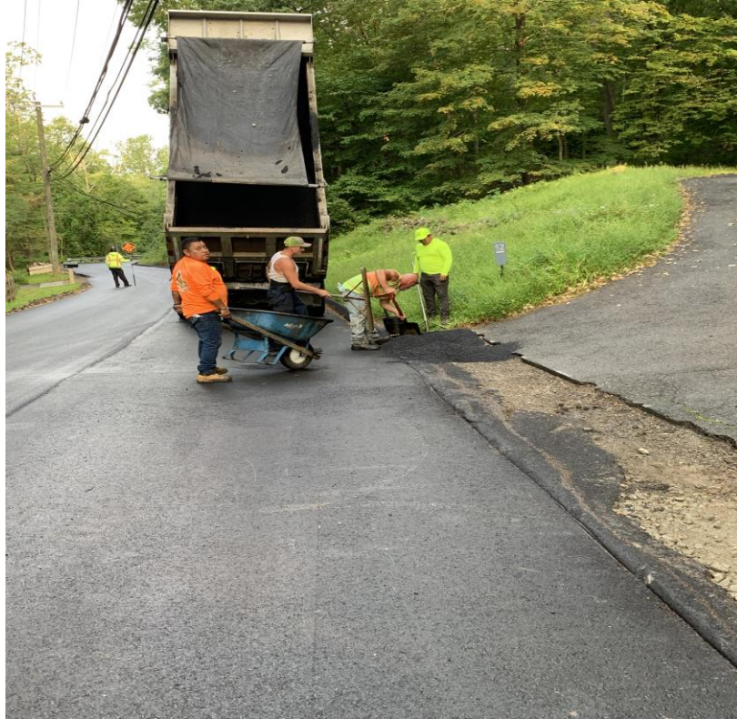
Replacing driveway aprons
