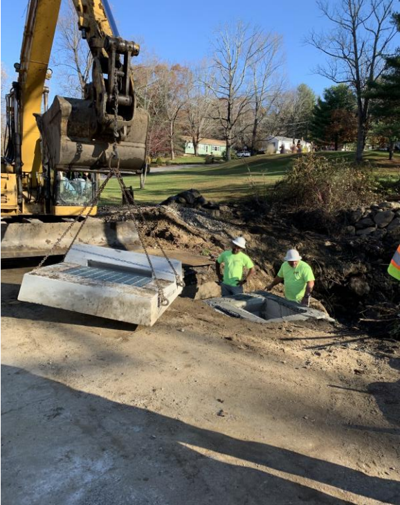
Replacing catch basin tops
