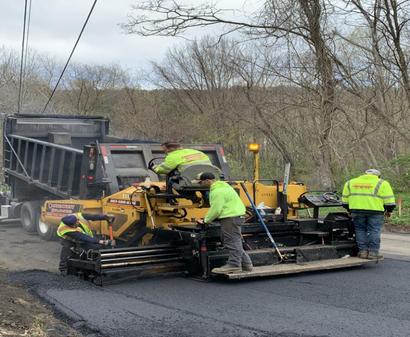
Paving base course
