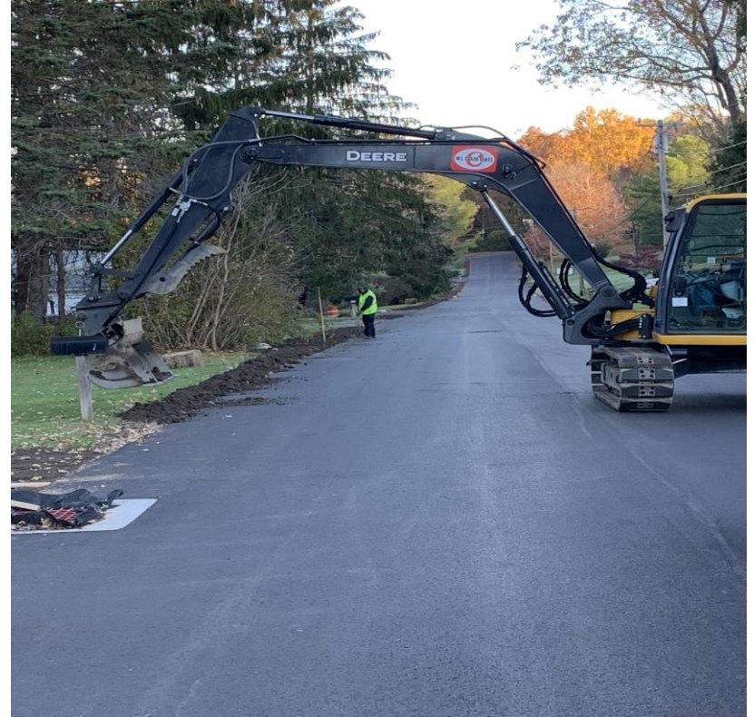
Backfilling edge of newly paved road
