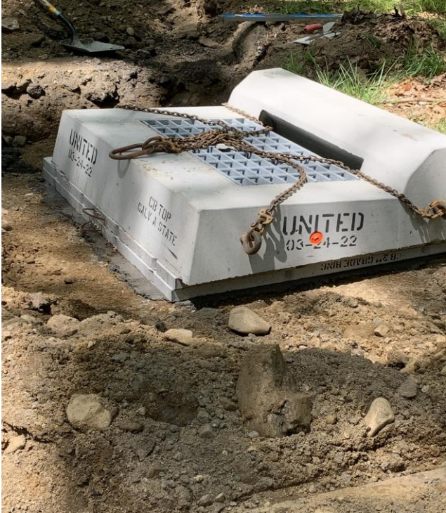
Replacing catch basin tops
