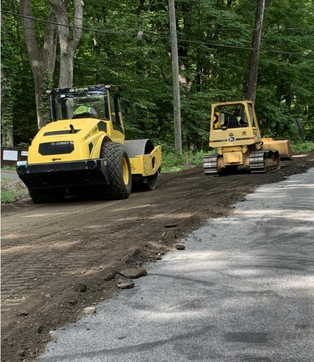
Rough grading & Compacting
