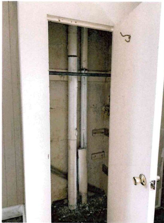
Photo 27: 1 st Floor Room 3 – ACM air cell pipe insulation and associated debris in closet shown.
