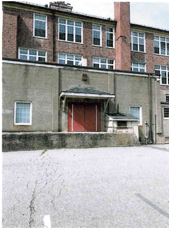
Photo 9: Lower slate (hip) roof and lower shed roof with black/gray caulking compound identified as ACM.
