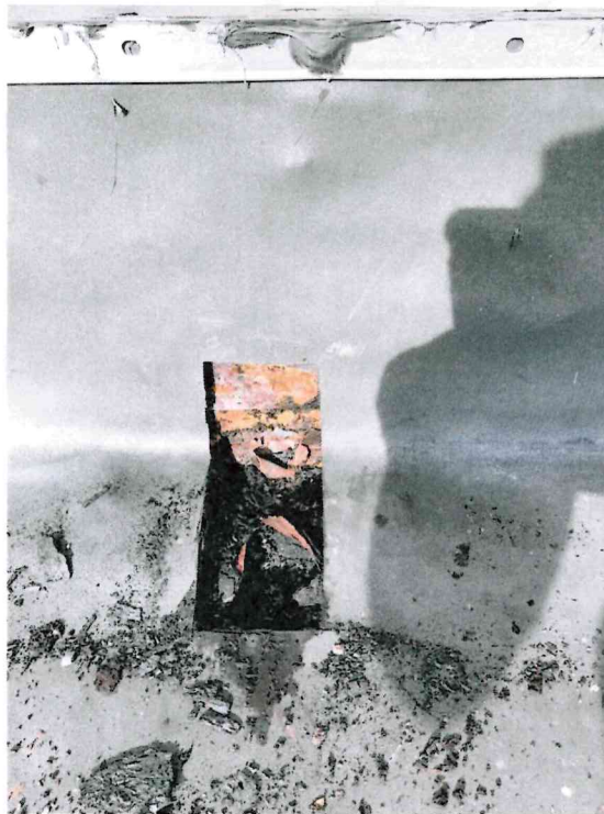
Photo 6: Upper flat roof flashing – Black tar/roof cement wall flashing over copper flashing identified as ACM.
