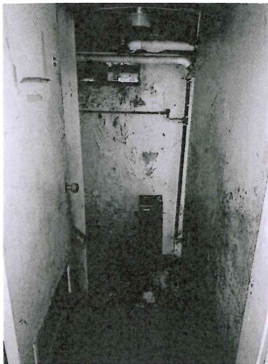
Photo 19: Basement – Northern men’s bathroom. Light fixture with asbestos containing paper, original metal window with asbestos containing caulking and glazing compounds, and 9”x9” red/brown asbestos containing floor tiles shown.
