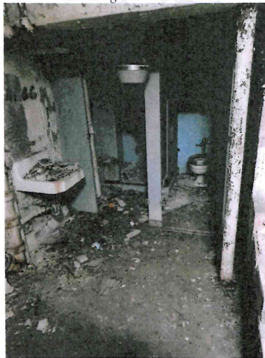
Photo 20: Basement – Southern (women’s) bathroom. Light fixture with asbestos containing paper, and 9”x9” red/brown asbestos containing floor tiles shown.
