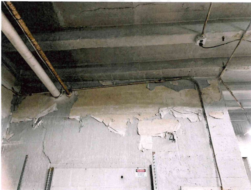
Photo 14: Basement Boiler Room – Silver paint identified as ACM shown.
