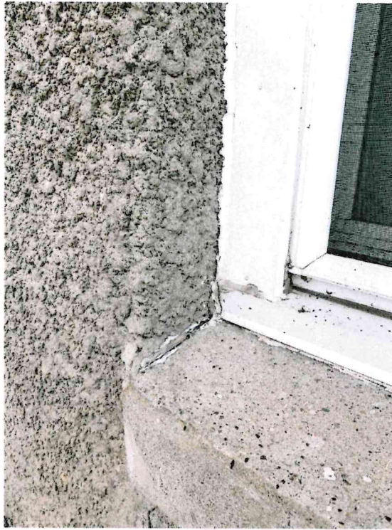
Photo 13: Typical residual asbestos containing caulking compound observed at new vinyl replacement windows (sampled at sill)
