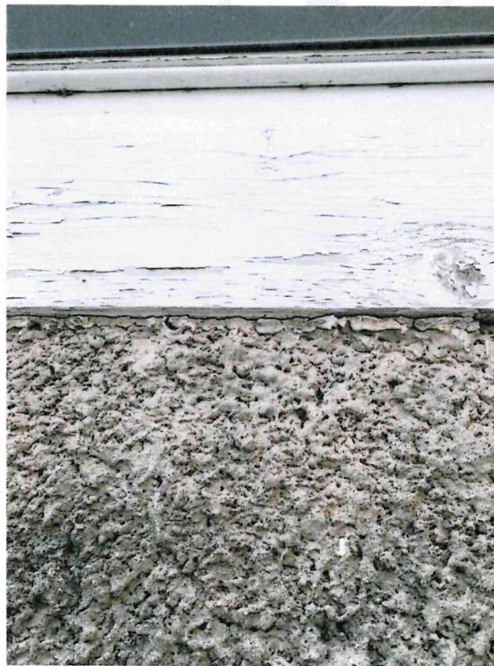
Photo 12: White caulking compound identified as ACM along upper flat roof fascia board.
