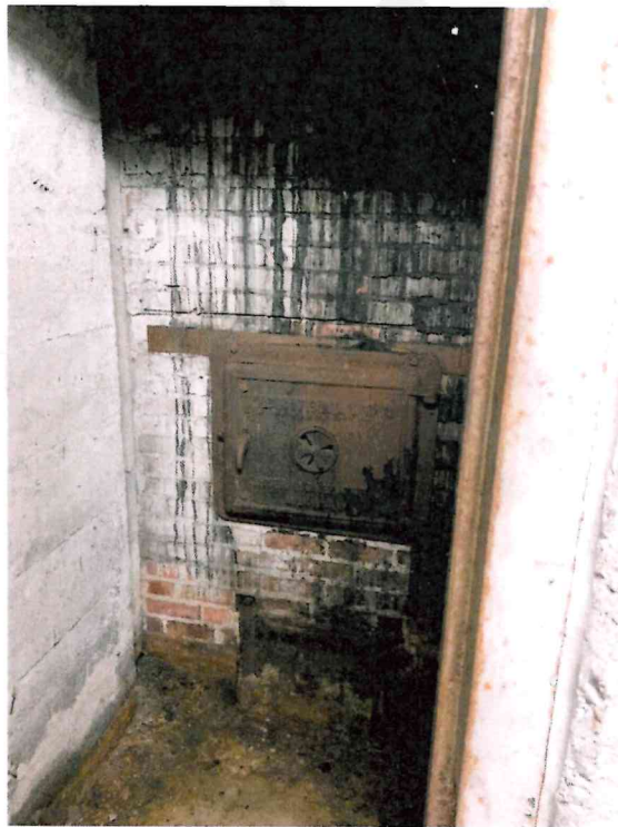
Photo 16: Basement Boiler Room – Incinerator with assumed internal ACM components shown.
