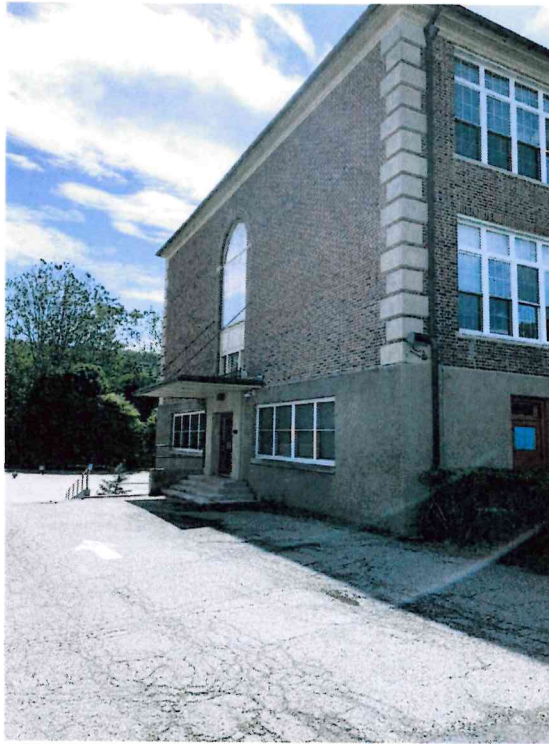
Photo 3: Site building northern elevation — Residual exterior window caulking compound identified as ACM possibly located at all windows including new vinyl replacement windows.
