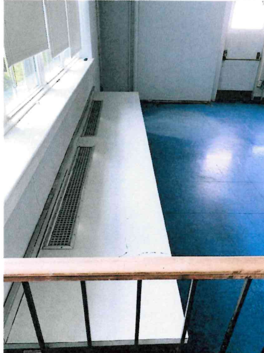
Photo 32: 1 st Floor Room 4 (southwest) – Cement board (assumed ACM) observed at back of cabinet.
