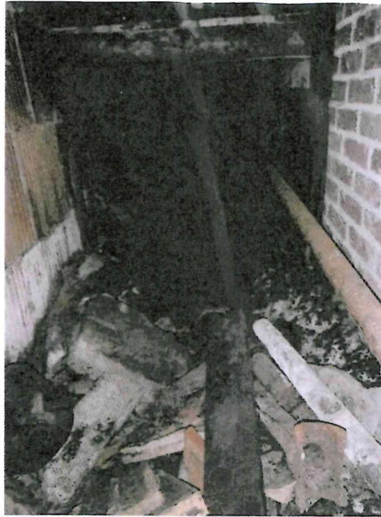
Photo 17: Basement northern tunnel system. Debris with potential buried ACM shown.
