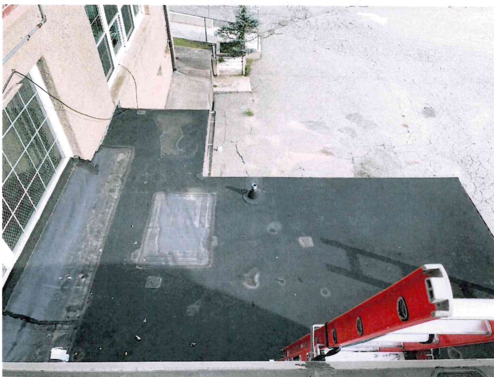
Photo 8: Lower flat roof (north end). Roof cement over flashing (repair shown below original windowsill) identified as ACM.
