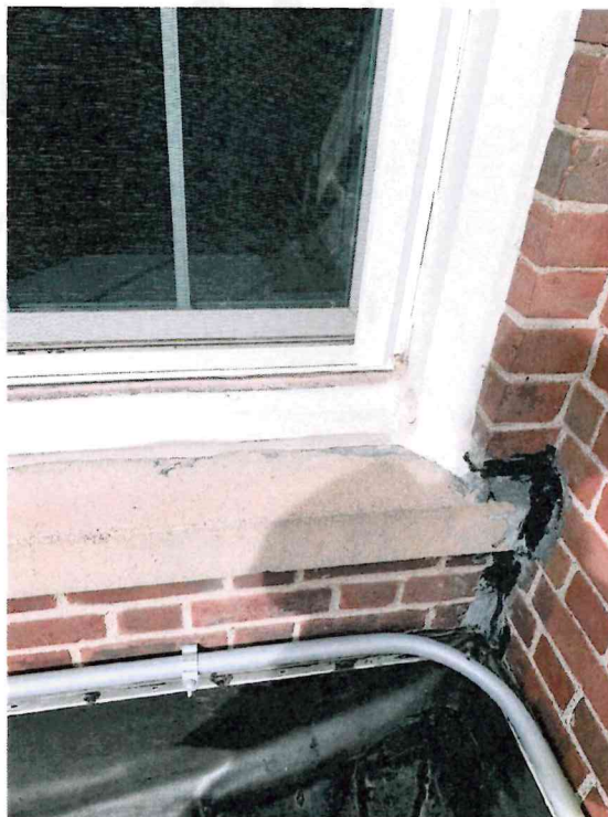
Photo 10: Black/gray caulking compound identified as ACM on brick wall at upper flat roof.
