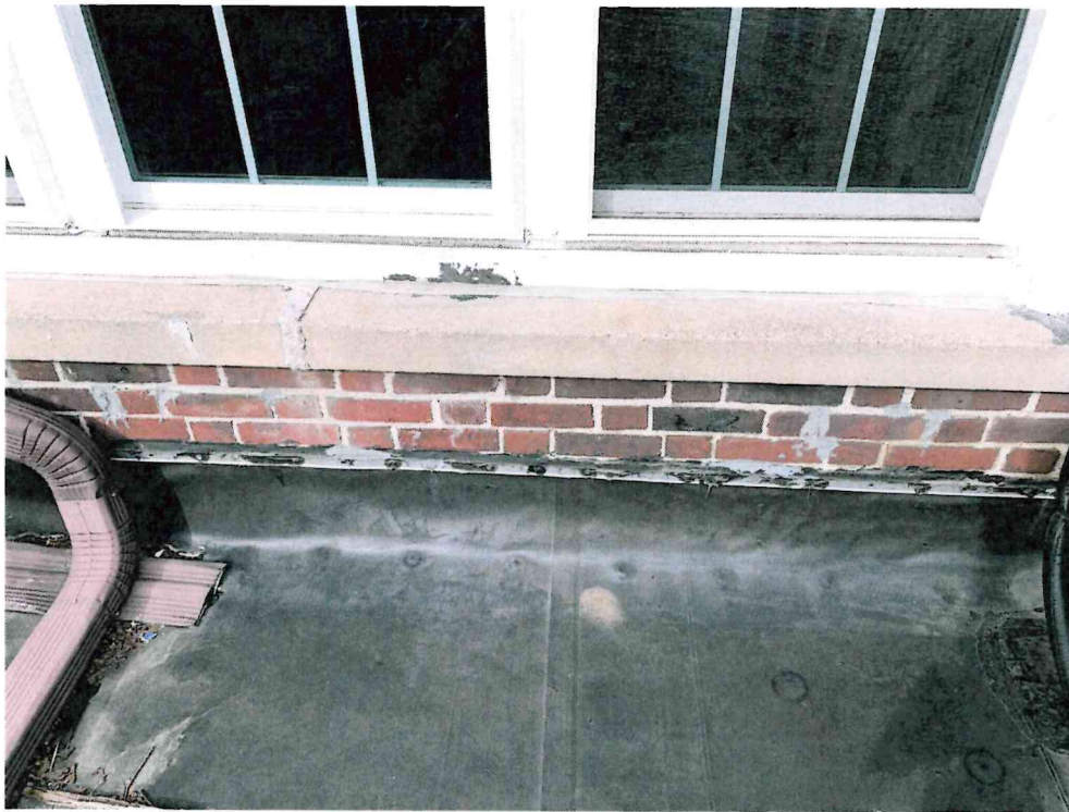
Photo 11: Black/gray caulking compound identified as ACM on brick wall at upper flat roof.
