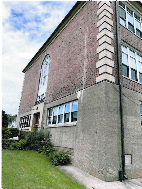
Photo 4: Site building southern elevation — Residual exterior window caulking compound identified as ACM possibly located at all windows including new vinyl replacement windows.
