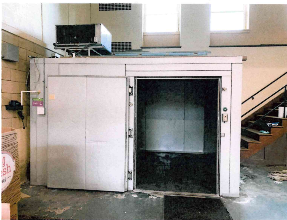
Photo 26: Walk-in freezer located in the Gym. Interior caulk and insulation assumed ACM.
