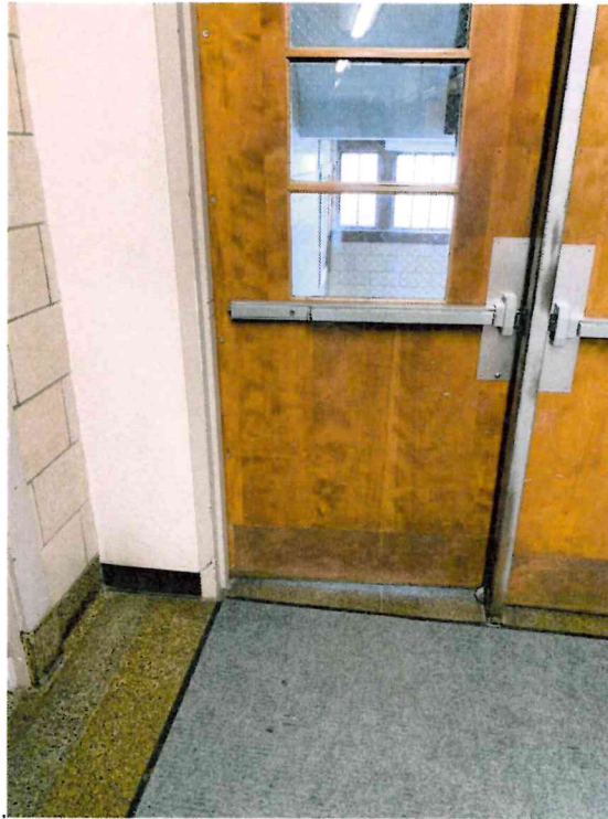
Photo 33: 2 nd Floor Hallway – 4” cove base molding with possible residual asbestos containing black adhesive shown.
