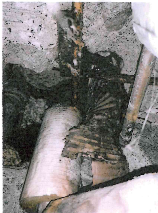
Photo 18: Basement northern tunnel system – Location of air cell pipe insulation (not visible in photo) and suspect corrugated cardboard at northeastern ceiling shown.
