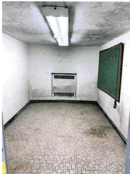
Photo 24: Lower level northwest storage storage/former shower (northwest). Gypsum/joint compound wall system with joint compound identified as <1% asbestos containing and cove base molding with possible residual asbestos containing black adhesive shown.
