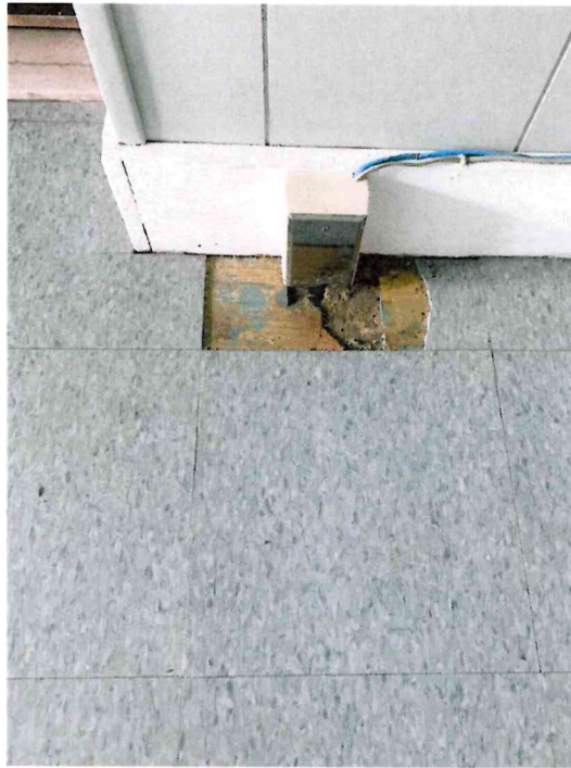
Photo 31: 1 st Floor Room 3 (southeast) – Blue tile below light blue 12x12 mottled vinyl floor tile identified as ACM (located on brown/tan 9x9 and associated mastic also identified as ACM).
