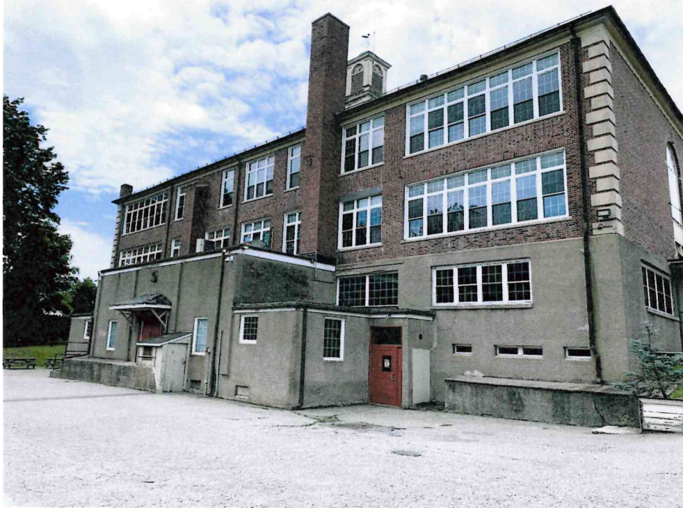
Photo 2: Site building rear entrances (eastern elevation) – Residual exterior window caulking compound identified as ACM possibly located at all windows including new vinyl replacement windows.
