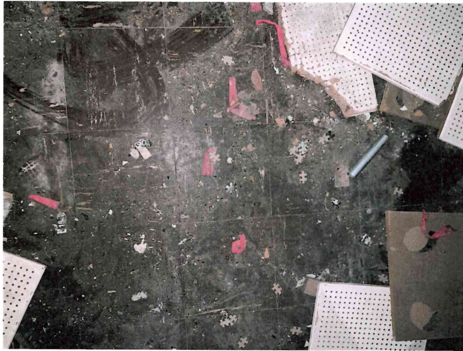
Photo 21: Basement – Northern (men's) bathroom. 9"x9" red/brown asbestos containing floor tiles shown.
