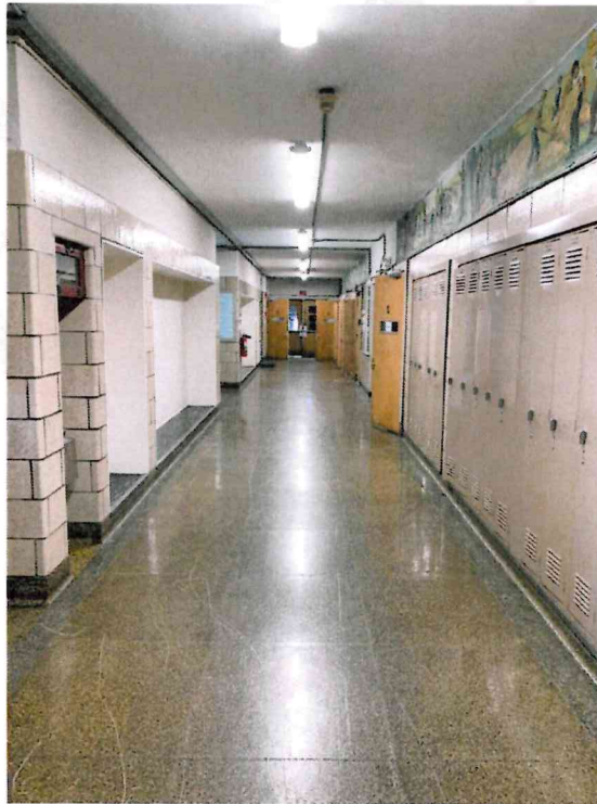
Photo 34: 2 nd Floor Hallway – 9”x9” Black vinyl floor tile at former locker nooks identified as ACM. Associated black mastic none detected for asbestos content.
