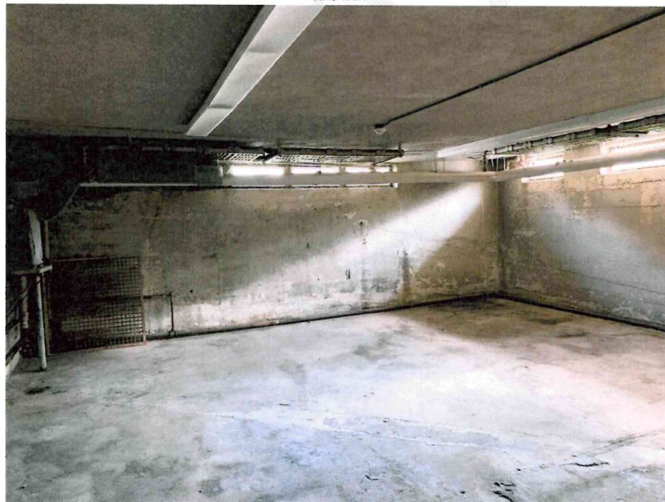
Photo 22: Lower-level mechanical room (northeast) - Ventilation system with white cloth vibration dampeners, silver paint on walls and ceiling (assumed ACM) shown and new vinyl replacement windows with possible residual ACM caulk shown.
