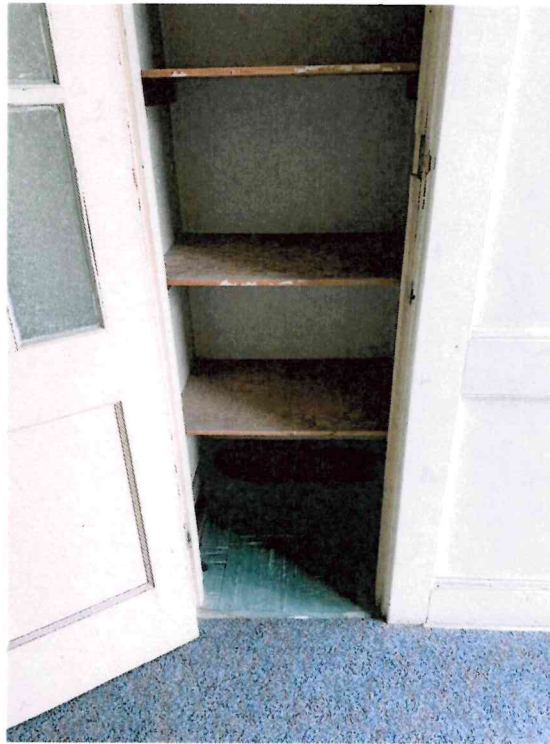
Photo 35: 2 nd Floor Copy Room – Asbestos containing 9"x9" green floor tile and associated black mastic located in closet and below carpet.
