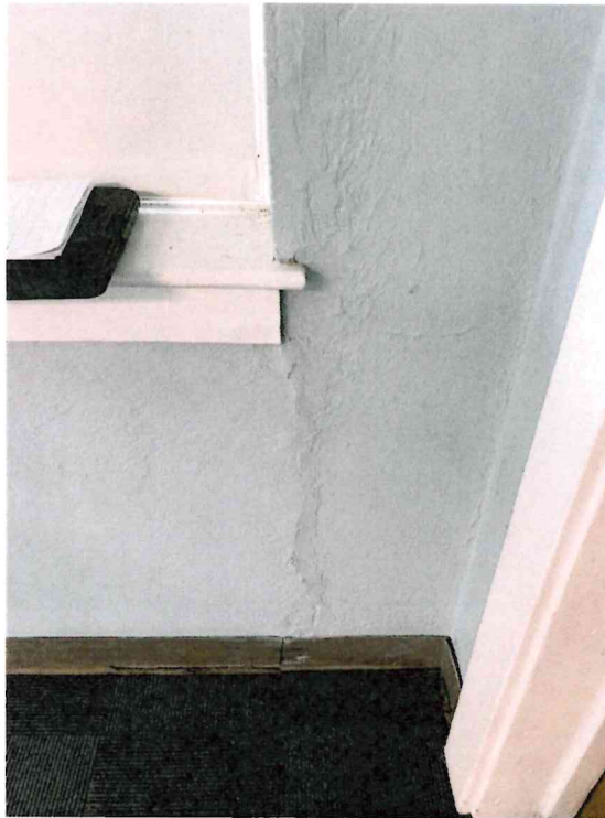
Photo 29: 1 st Floor Room 2 (northwest) – Typical 4” brown cove base molding with possible residual asbestos-containing black adhesive.
