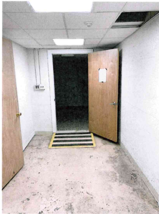
Photo 23: Lower level northwest storage entry/vestibule - Gypsum/joint compound wall system (at right) with joint compound identified as <1% asbestos containing and cove base molding with possible residual asbestos containing black adhesive shown.
