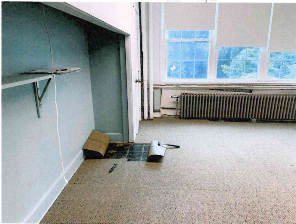
Photo 36: 2 nd Floor Room 5 – Residual black mastic located below carpet on hardwood identified as <1% asbestos containing.
